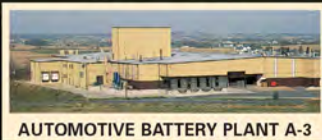
AUTOMOTIVE BATTERY PLANT A-3
