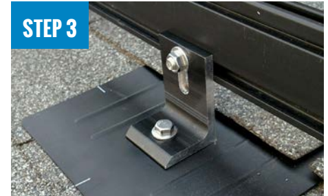
ATTACH L-FOOT TO RAIL
