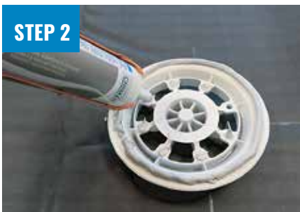
APPLY CHEMLINK M1 SEALANT
